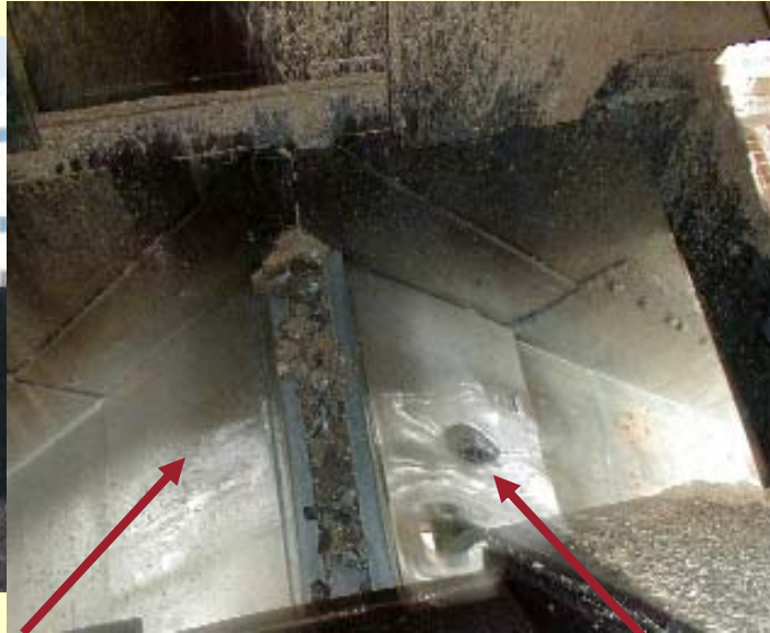
TRIP (field test on separator) standard
