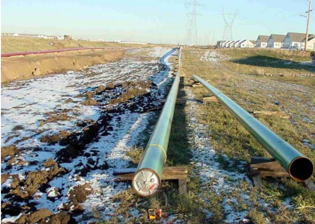
FIGURE 5: Various Length Pipe Sections on Skids in HVAC ROW
