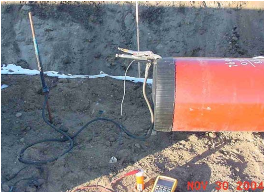
FIGURE 6: Capacitive Coupled AC Temporary Grounding Mitigation
