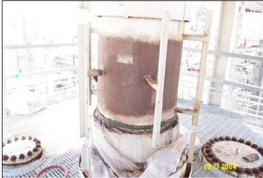
FIGURE 28 – Surface preparation of gas dryer unit prior to application of TMIC.
