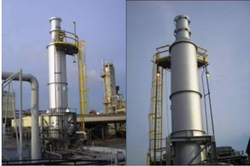
FIGURE 22 – Incinerator after remediation and TMIC application.
