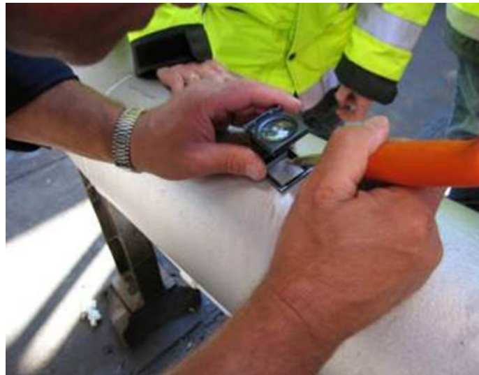
FIGURE 25 – Sweden Refinery Piping – condition of TMIC after 2.5 years service.
