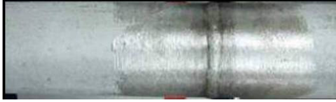
FIGURE 14 – Welded pipe joint after surface preparation to SSPC-SP11.
