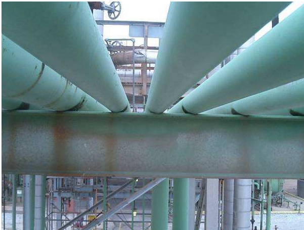
FIGURE 2 – Simple Pipe Supports
