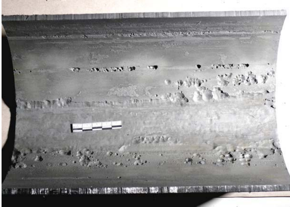
FIGURE 5 - Band of General Wall Loss (50% Loss) and Isolated Pitting (25-30% Loss) adjacent to external grooves in the HDPE liner
