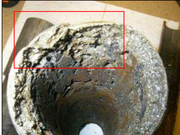
FIGURE 7 - Downhole corroded tubing showing characteristic ductile failure
